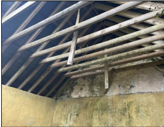
Plate 4-24 Timber support beams and felt lining inside Structure 2, which can provide shelter for roosting bats.
