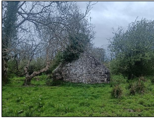
Plate 3-1 Northeast aspect of Structure No. 3
