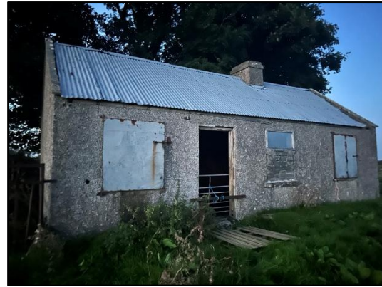
Plate 3-2 Southern aspect of Structure No. 1
